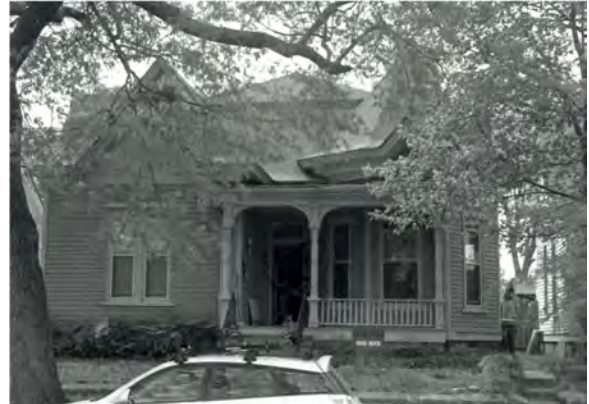
Figure 9: 908 S. Rock St., photo courtesy of Arkansas Architectural Resources Form, 2007.
