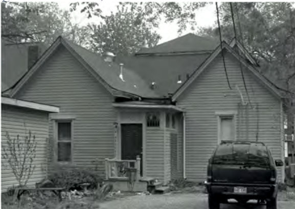
Figure 10: 908 S. Rock St., photo courtesy of Arkansas Architectural Resources Form, 2007.
